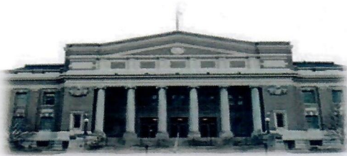
Franklin County Memorial Hall
